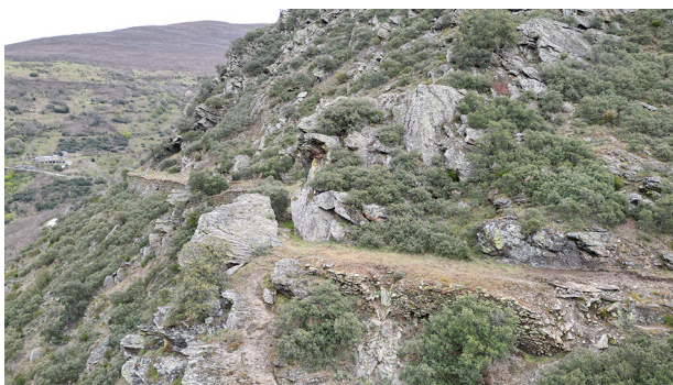
Fig. 4 Roman hydraulic system. Trace of channel to Las Médulas, cut into the rock and featuring a dry-stone retaining wall.
