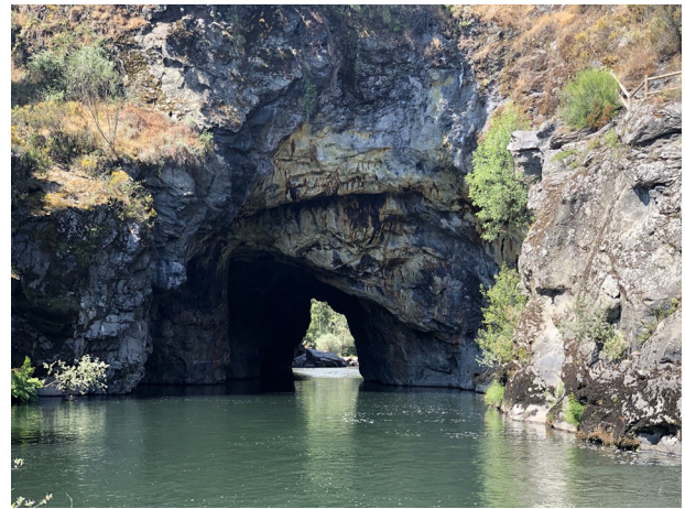
Fig. 7 Anthropogenic river course modification. Montefurado tunnel (Montefurado, Lugo), built to divert the river to exploit the gold-bearing sands along the entire meander of the Sil River.
