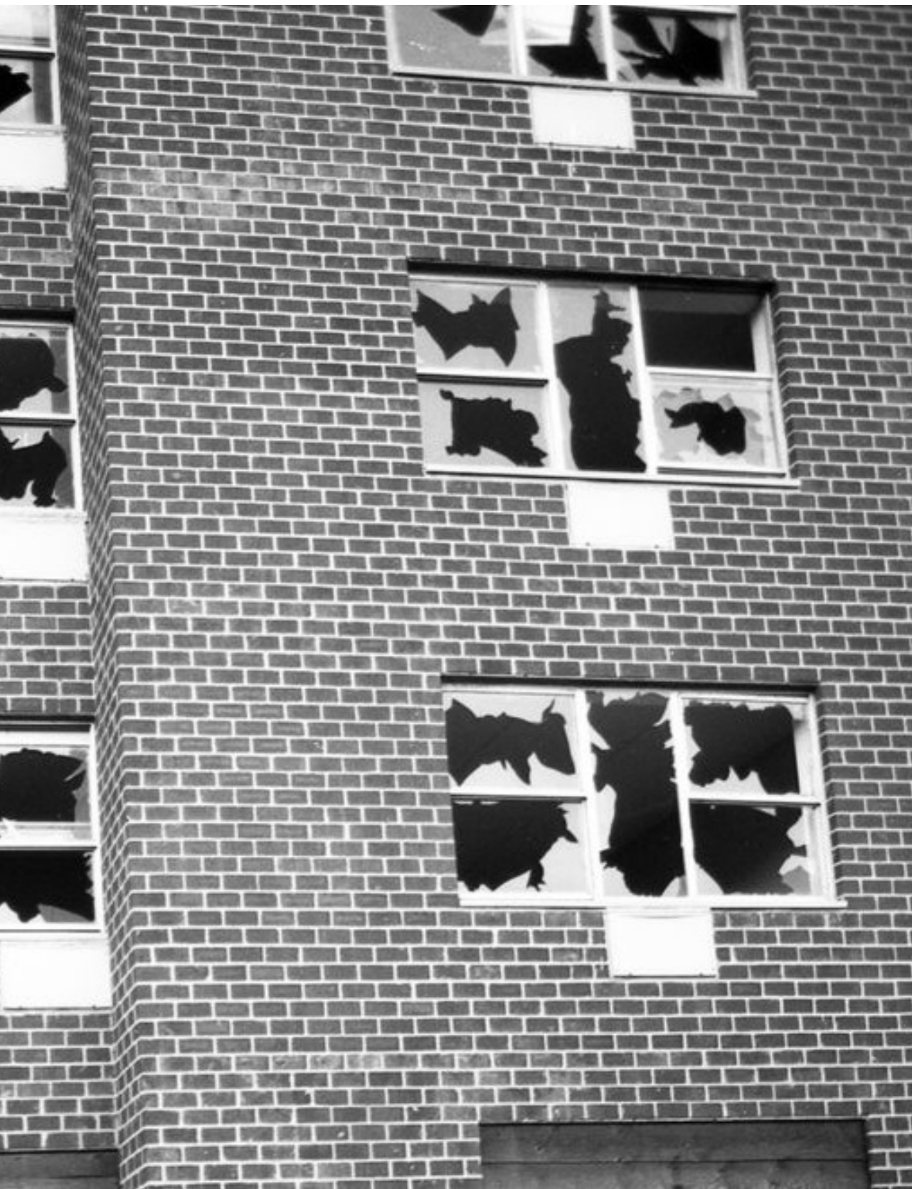
Gordon Matta-Clark Window Blow-Out 1976 (406 x 559 mm)
